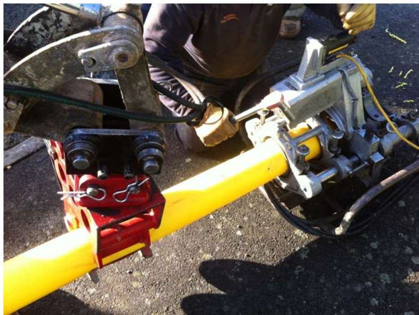
Image 15, Mini Pipe Handler and butt fusion machine.
