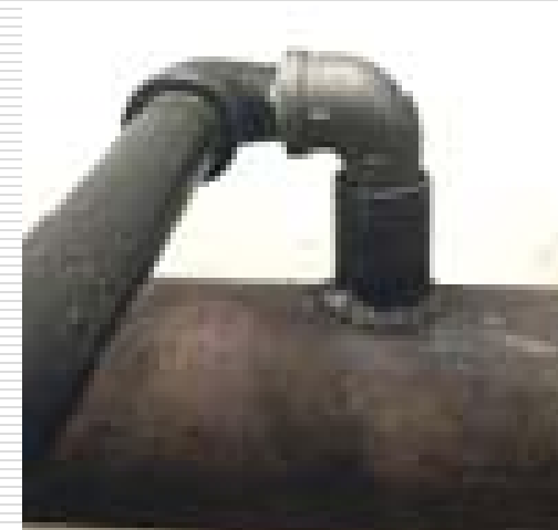
Male x Female Elbow threaded into a coupling
