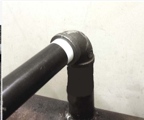
Female x Female Elbow on a TOE nipple
