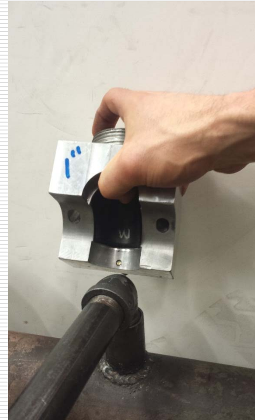
Fit Elbow Housing.
