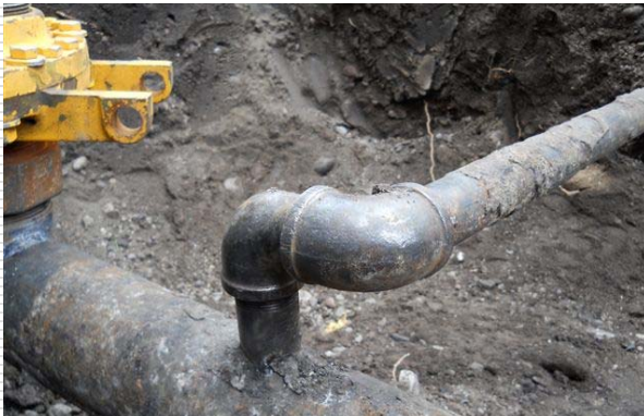
Female x Male Elbow on a TOE nipple
