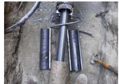
Circumferential Cutter Module
