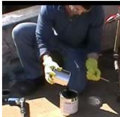
Pour the entire contents of the Part B can into Part A can.
