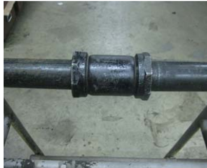
Typical Dresser Style 90 / NORMAC Compression Coupling shown.
