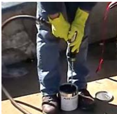
Hold the part B can between your feet so it cannot spin and mix vigorously for 1 minute using a Jiffy mixer in a 500 rpm geared air drill.
