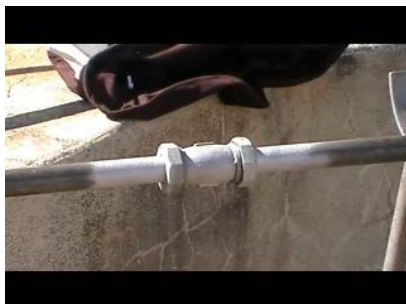
Grit blasting completed.
