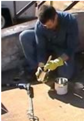
Scrape any solids from the bottom of the Part B can and mix with the paint paddle.
