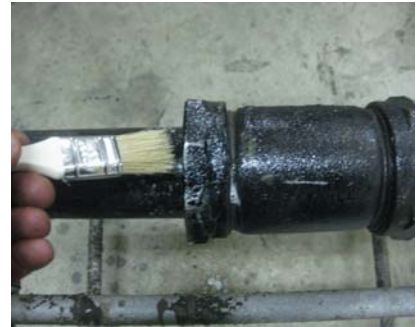
Soap test for leaks.
