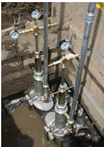
Simple Double Block and Bleed Operation
