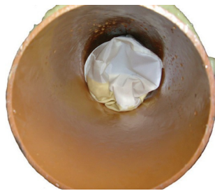
A.) Bag in a pipe during the start of expansion.
