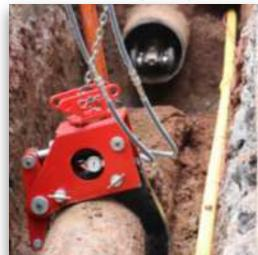
**Safe:**The squeezing action is controlled remotely from the cab or road surface to gently break the pipe, preventing flying debris.
