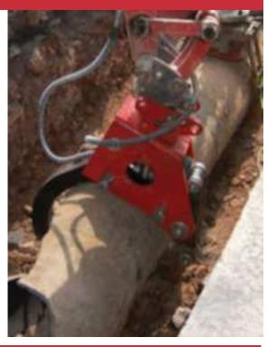
Note: The tool does not break a clean edge. To do that, use a snap cutter or 4-wheel cutter to score or cut, then use the Cracker to remove the middle. The cast iron pipe middle section will not move if only the two ends cut. The center is smashed out with a sledgehammer.
