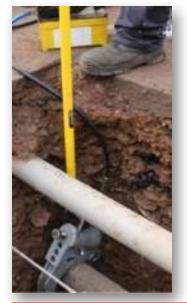
Break out 3", 4" and 6" cast iron pipe in a couple of minutes from the surface.
