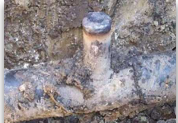
Weld around edges to seal pipe.
