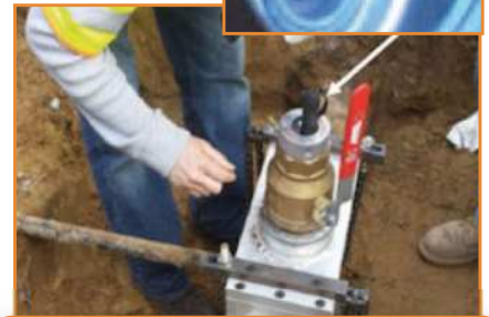
Sight glass view of service tee main hole to plug off.
