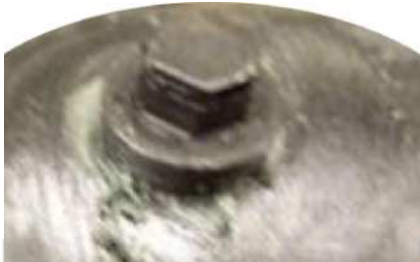
Tighten into pipe to plug the hole.
