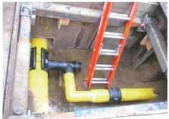
Figure 2 – Supraflow Excavation Fit
