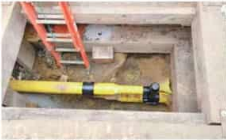
Figure 8 – Site 2: Main Extension for New Service
