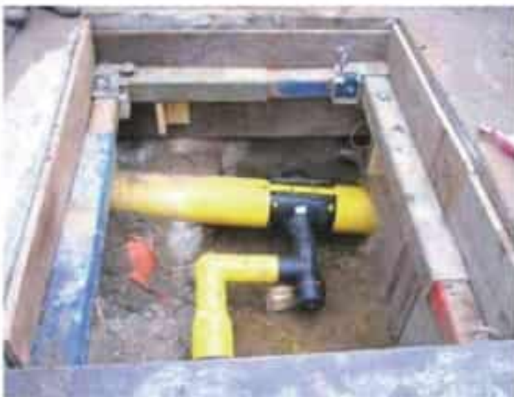
Figure 9 – Site 3: Horizontal Service Installed in an Inclined Main
