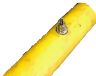
(Photo 24-A) – Rubber Plug in main
